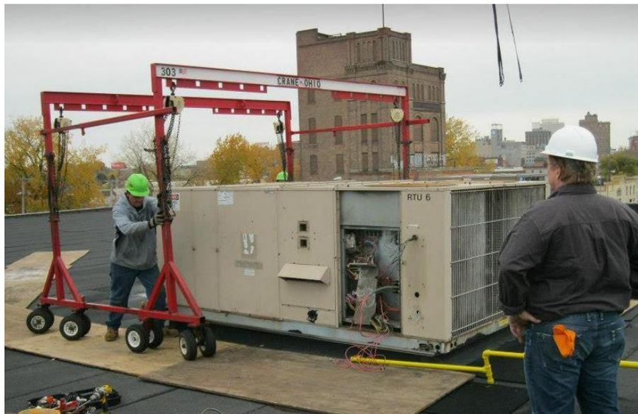
*The gantry slides into place to lift the old unit as a rooftop package unit is replaced*
