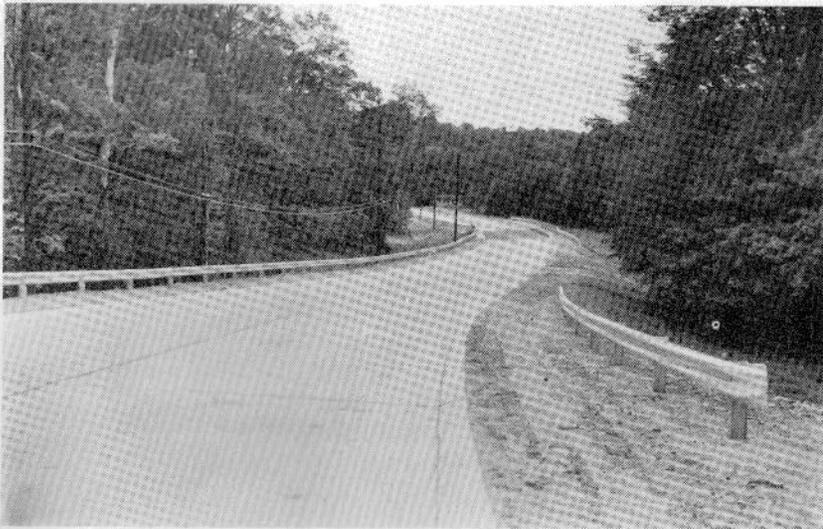
**THE NEW HARRIS ROAD BRIDGE HIGHWAY:** In addition to a new bridge 1200 feet of highway was constructed, guard rails installed for safety, the road was straightened thereby eliminating dangerous curves, and culverts installed to insure proper drainage.
